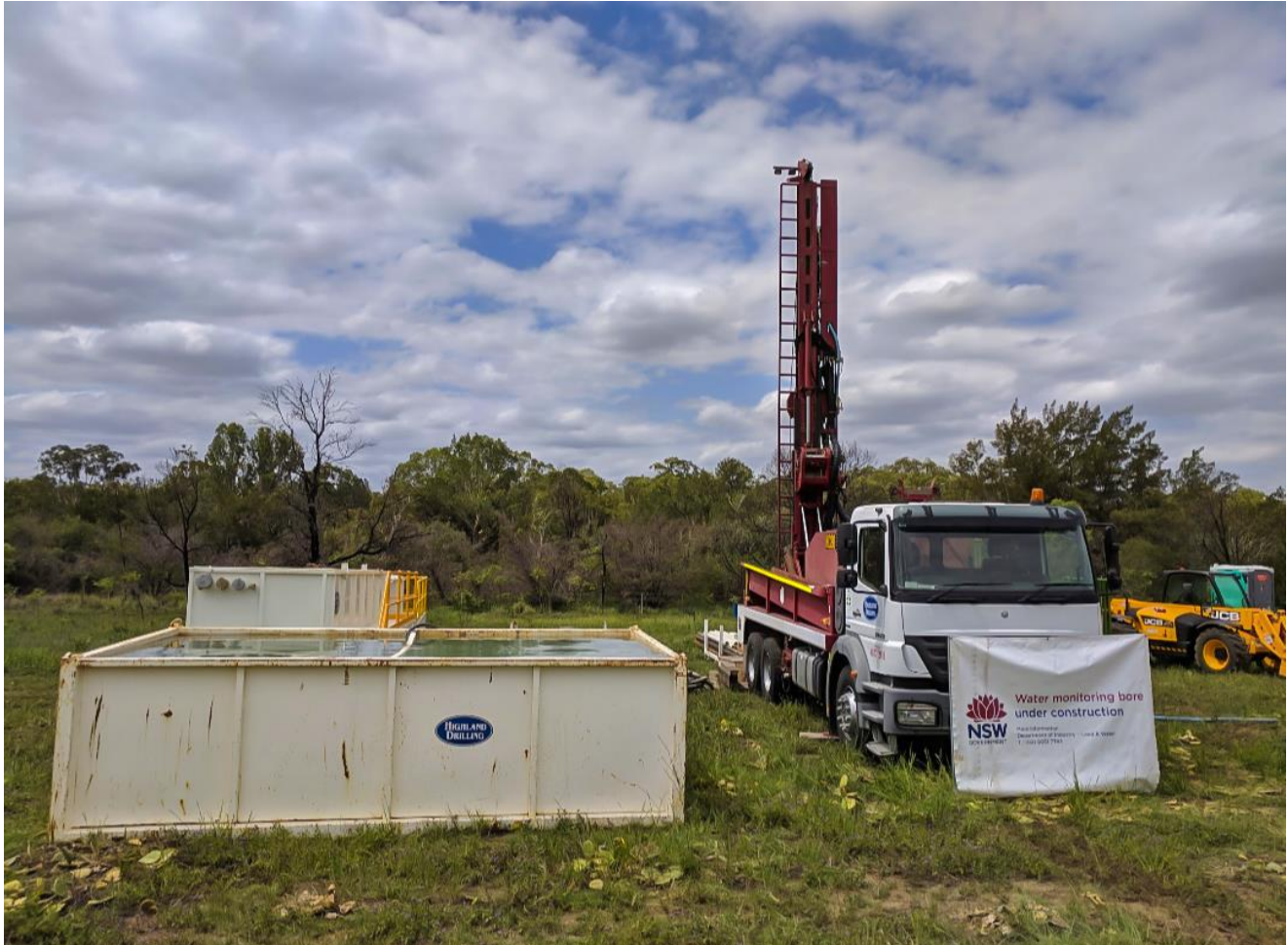
Figure 5 - Groundwater monitor bore drilling. Credit: Jake Turi / EMM
