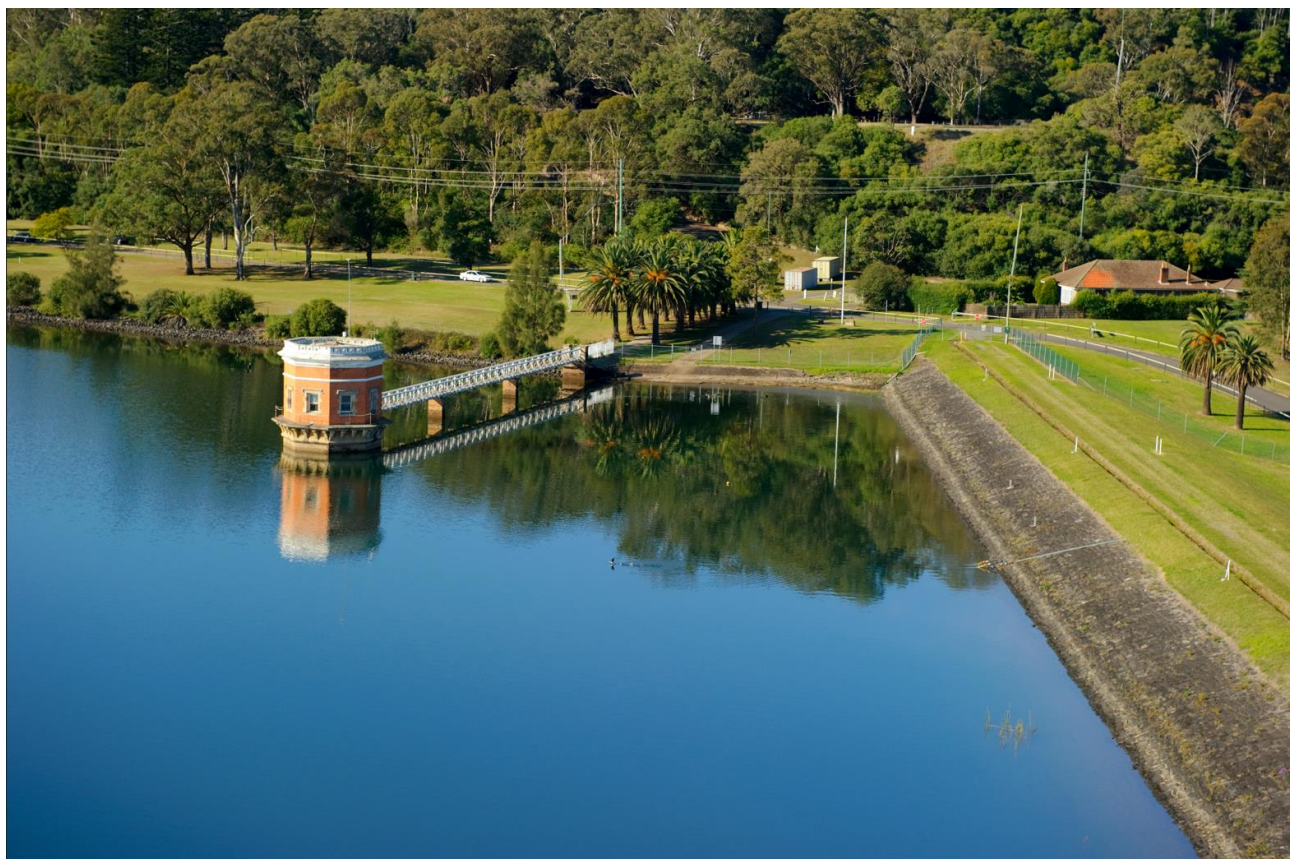
Figure 1. Prospect Reservoir featuring the submerged pumping station (source: WaterNSW)
