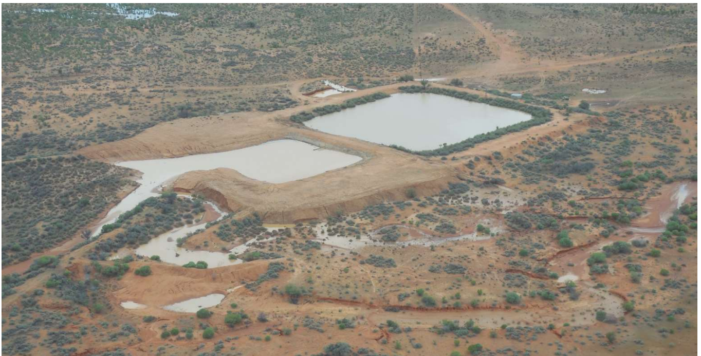
Figure 1: typical excavated earth dam in western NSW.
