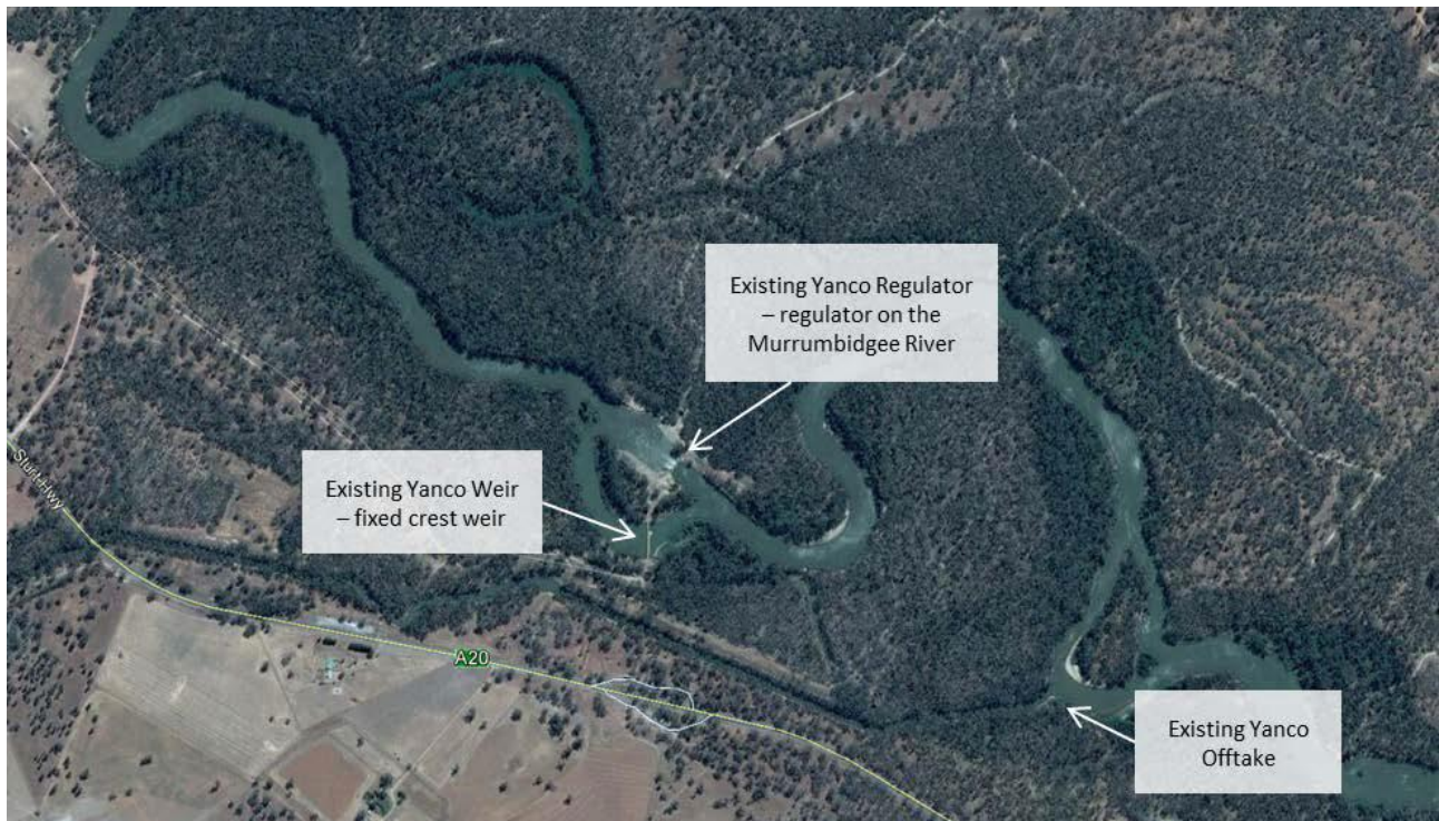
Figure 4 Existing Yanco Creek Offtake infrastructure (source: DPE April 2022)
