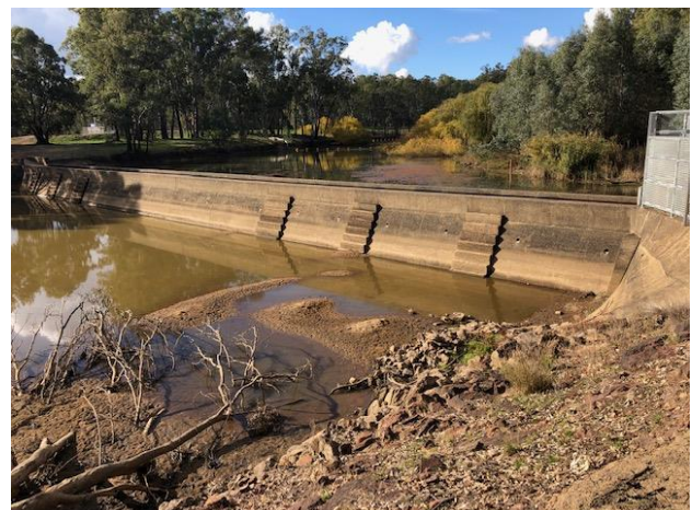
Figure 6 Yanco Weir (Fixed Crest Weir)
