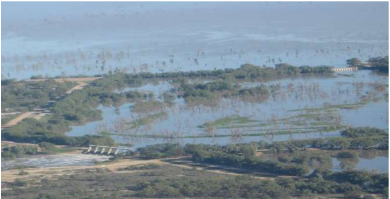
Main Weir (bottom left) – the start of the Lower Darling River.
