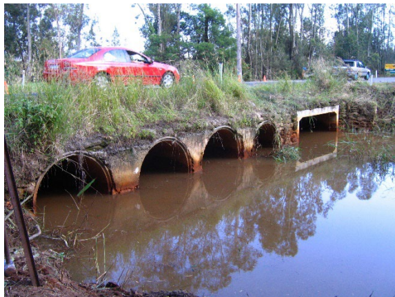
Figure 30. Major infrastructure in place to accommodate drainage systems
