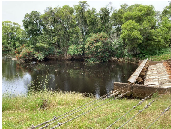
Figure 40. Large floodgates releasing a high volume of de-oxygenated blackwater into the river, overwhelming the downstream capacity to dilute the impacts
