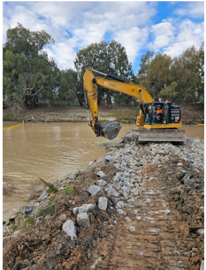
Figure 2: Excavator creating platform to support weir removal.
