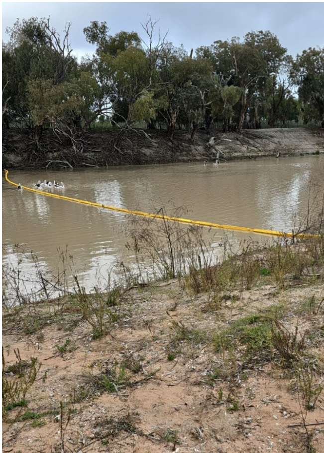
Figure 1: Yellow silt barrier crossing the span of the river.
