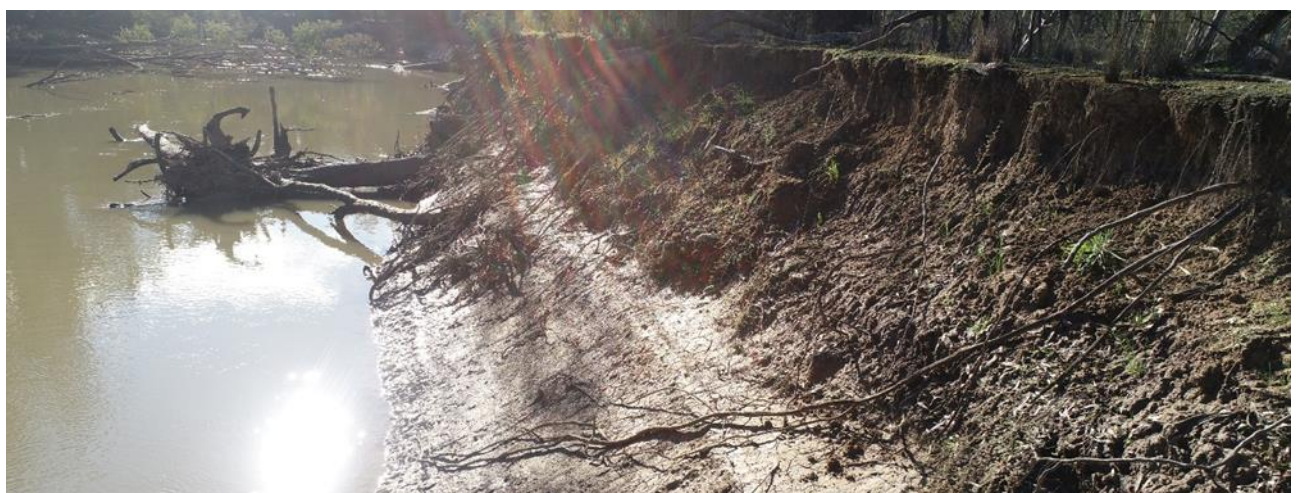
Figure 22 Mass failure of the bank on the Edward River (Watts et al, 2020)
