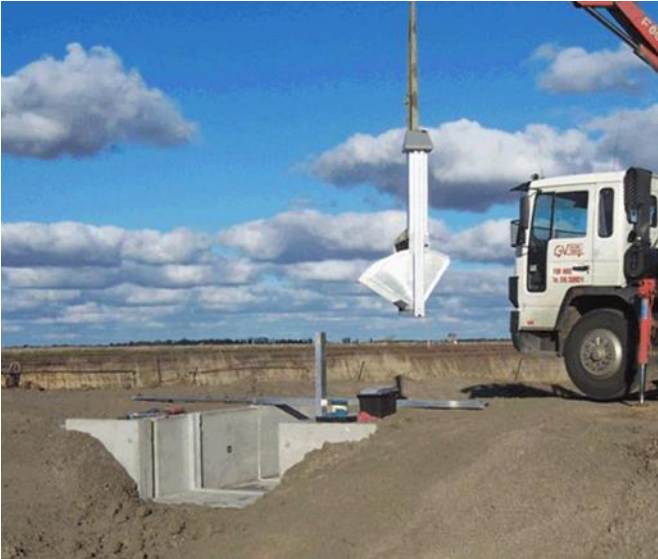
Figure 9. Installation of gate meter
