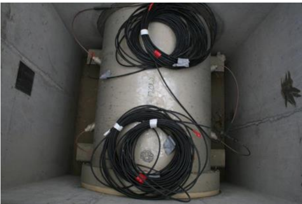
Figure 6. Example of a transit-time ultrasonic meter
