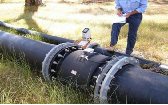
Figure 5. Example of an electromagnetic flow meter
