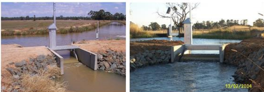
Figure 8. Example of gate-type meter in standard and large irrigation outlets
