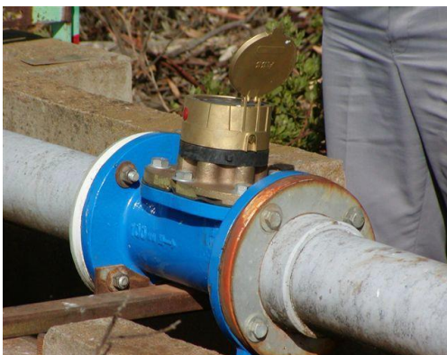
Figure 2. Examples of propeller-actuated meters
