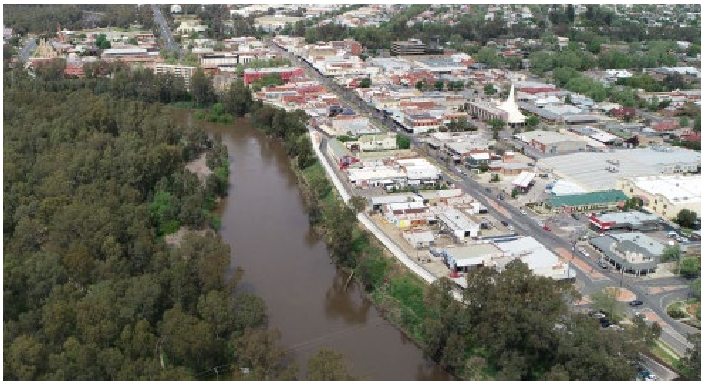
Wagga Wagga Murrumbidgee River levee bank
