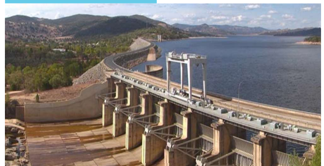
Wyangala Dam wall
