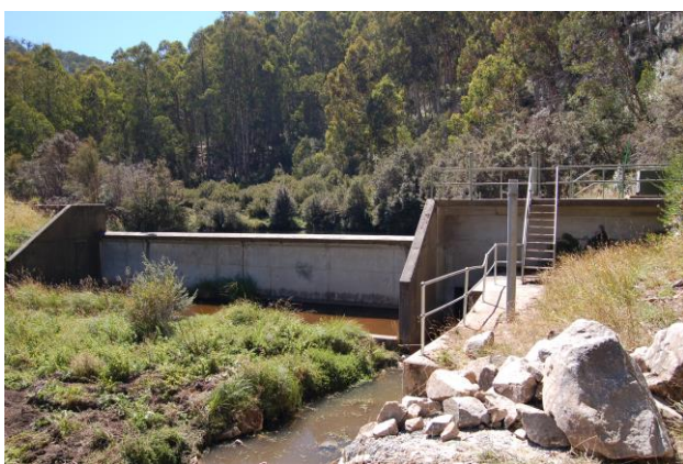
Middle Creek weir
