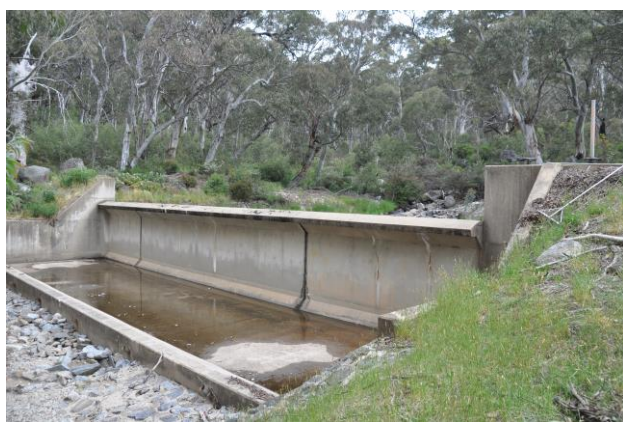
Diggers Creek weir
